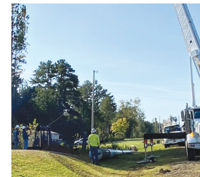
New Transmission pole installation in Polk County
