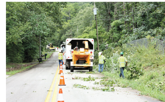
ROW contract crews cleaning up the large limbs with a portable chipper.
